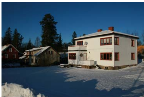
Villa i Gardermovegen
